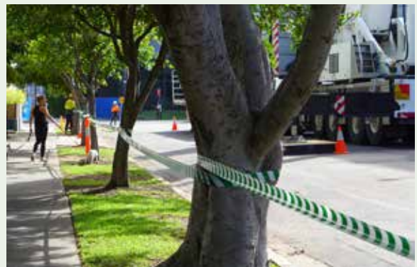
Figure 7: Appropriate barriers must be installed to isolate an approved work/crane operation area. In busy pedestrian areas such as the city-centre, metal barriers must be used.
