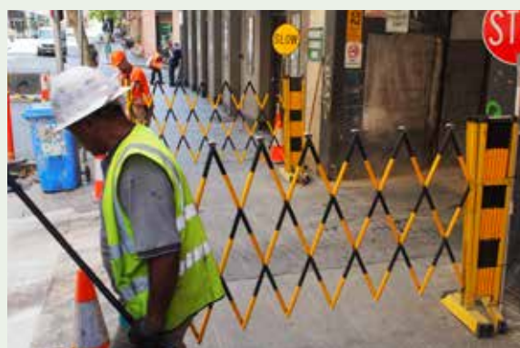
Figure 43: The effective control and safety of pedestrians and cyclists at truck access points is essential. This is particularly important in high volume pedestrian areas. The City will allow, and require, the use of manned concertina gates as a control measure .
