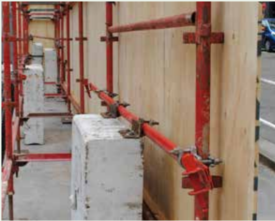
Figure 4.8: Scaffolding encapsulating a building undergoing demolition and later used as a hoarding site fence must be adequately counterweighted. Wind actions in the locality including potential extreme wind velocities from surrounding buildings must be considered by the person in control of a worksite and the scaffolding contractor. Excavated sites must also be protected using appropriate pedestrian and traffic barriers (see 2.13).
