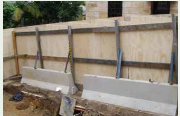
Figure 2.13: A Type-A hoarding braced to a concrete Jersey kerb and protecting an excavation.
