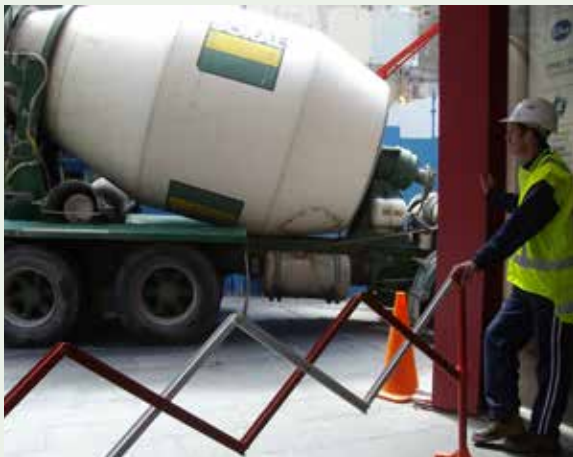
Figure 3.59: Concertina gates to control pedestrian and cyclist movement at truck access points are mandatory in the city-centre and in other busy pedestrian areas outside the city-centre. Gates must be provided on each side of vehicular crossings including cycleways . Specific approval of the City must be obtained before installation/usage.
