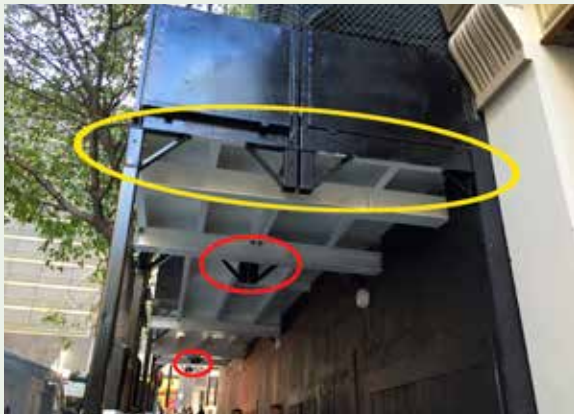
Figure 3.57: Example of a non-compliant design. Fascias must extend to cover the structural members in a single plane to allow graphics to extend over the entire surface (circled yellow). Note also that all structural members to the soffit of the deck are to be painted white.
