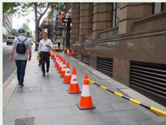
Figure 16(a): Temporary barricading must minimise impacts and maintain safe and convenient pedestrian passage. In some cases barricading will not be permitted during the peak pedestrian periods. In very busy areas such as shopping districts, works and barricading may need to be undertaken at night or on weekends.
