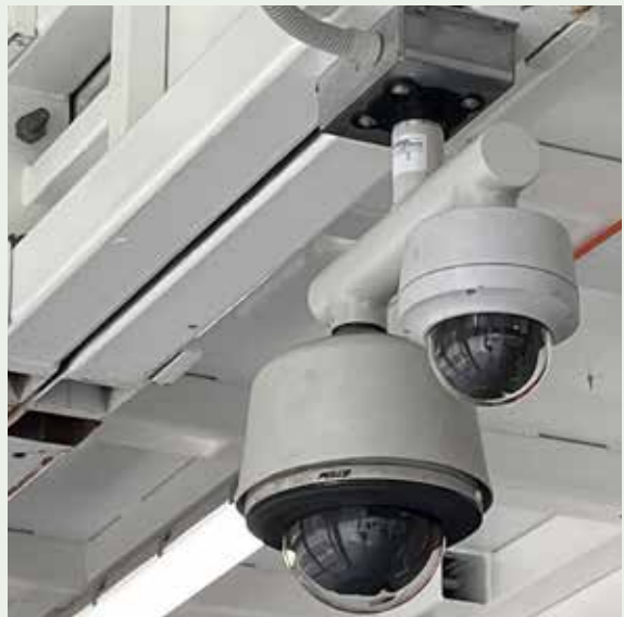
Figure 2.3: Sightlines from City -operated CCTV surveillance cameras must not be obstructed by temporary structures . Traffic monitoring cameras (and private property cameras required by a condition of development consent ) must also not be obstructed. Remounting the City's cameras beneath hoardings may be an acceptable solution. Refer to 2.17 for information on private CCTV surveillance cameras mounted on temporary structures .
