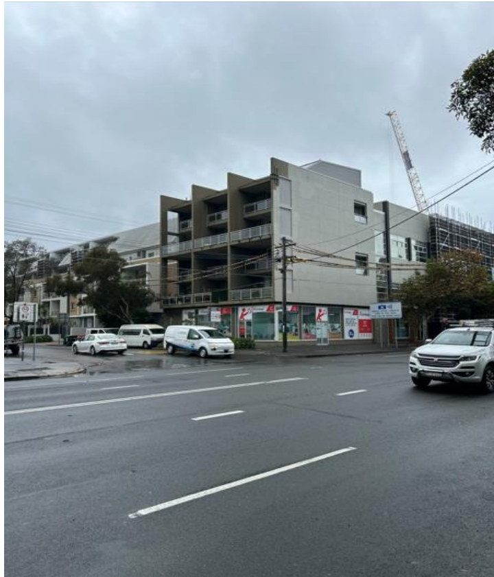
Figure 1: 4 Gillespie Avenue, Alexandria, viewed from the south-east
