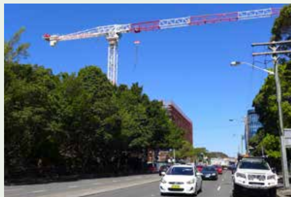
Figure 12: Approval under the Roads Act is required when any part of a hoisting device swings or operates over a road including encroachment under wind-vaning actions.
