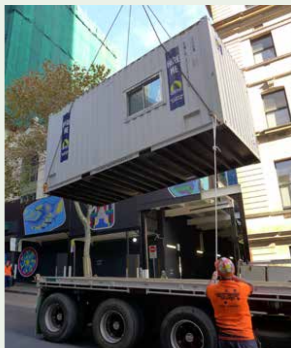
Figure 10: All hoisting operations must be carried out within the boundaries of a works zone or a temporarily closed traffic lane (to a height of at least 4.5 metres above the road surface ).
