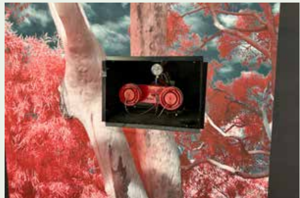
Figure 3.41: Fire brigade booster connections behind site fences must be kept available. Graphics fabric must be neatly trimmed/finished around openings.
