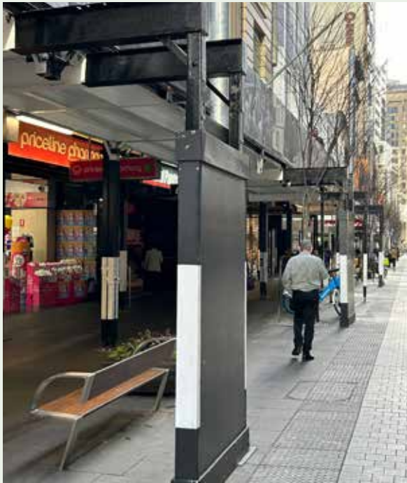
Figure 3.8: Exposed beams and other elements beyond the deck perimeter must be painted black.
