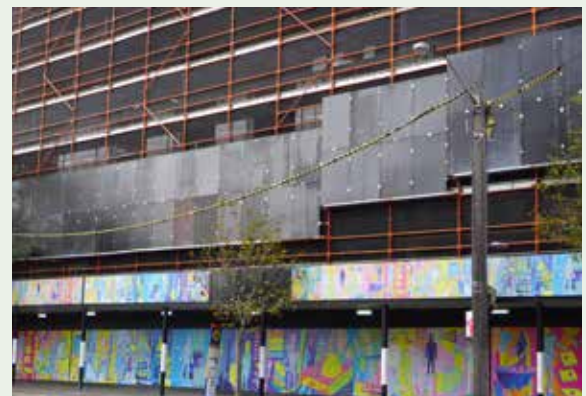
Figure 2.9: Where plywood sheeting is required to shield temporary structures from aerial electricity cables all sheeting must be painted in a colour and tone that matches the scaffolding containment mesh (see 'Note' below).
