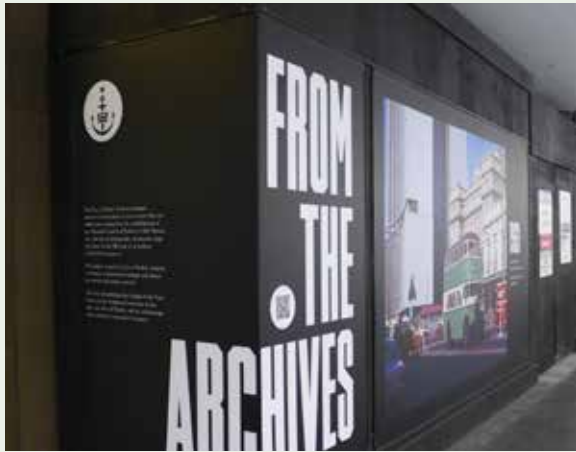
Figure 6.15: Where a hoarding depth is more than 0.5m, graphics must be displayed on the end panels. The printed fabric should be wrapped on the corners (to avoid double vertical sail-tracking). Where a historic display is required, the 'From the Archives' panel can be appropriately wrapped on the corner as shown in this figure.
