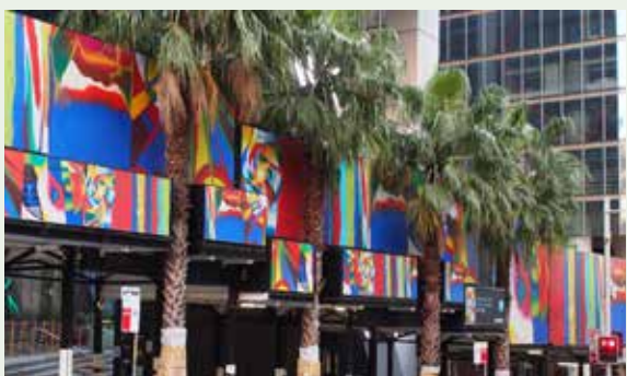
Figure 3.67: Hoardings must be designed to minimise impacts on tree canopies and maintain clear pedestrian passage. This can be achieved by designing a system of strategically placed columns and bridging beams (see also Figure 3.63 ).
