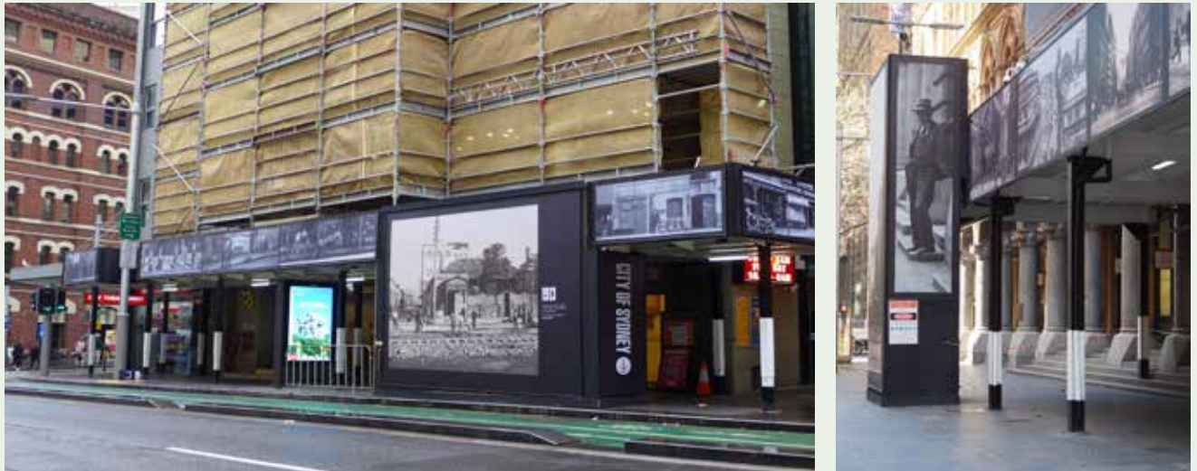
Figure 3.53: Access stairs must be fully enclosed and appropriately finished to allow the display of graphics in a single panel at the kerbside and on other surfaces with the exception of the access door and panel. as required by Part 06 .
